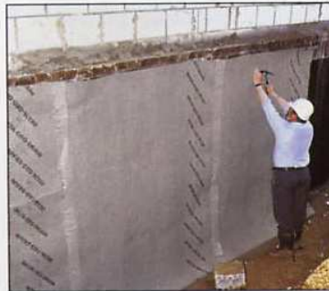
The DELTA-GEO-DRAIN protection and drainage system is laid in rolls with the smooth side (slip-layer membrane) facing the brickwork and the applied geotextile facing the soil.
