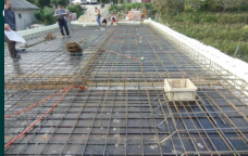
reinforcement during placement
