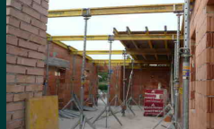
formwork during installation
