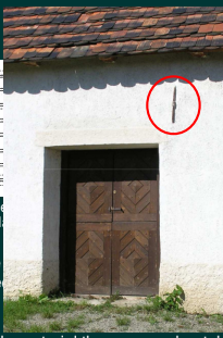
anchorage of a beam head to walled iron plate walling the beam head (underlayment, ventilation)
