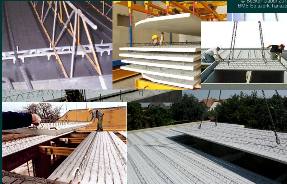
formwork panels prefabricated floors - plank floors
