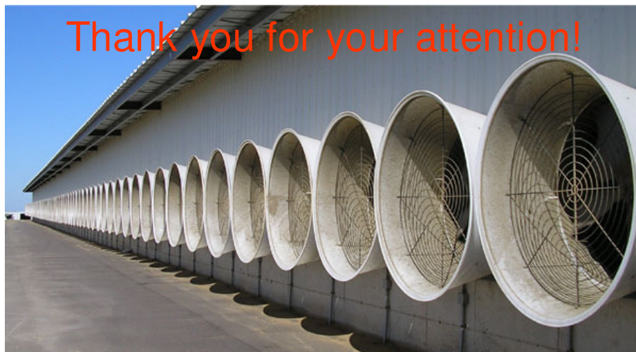
Exhaust fans on a cross-ventilated barn by Kevin Janni – University of Minnesota
