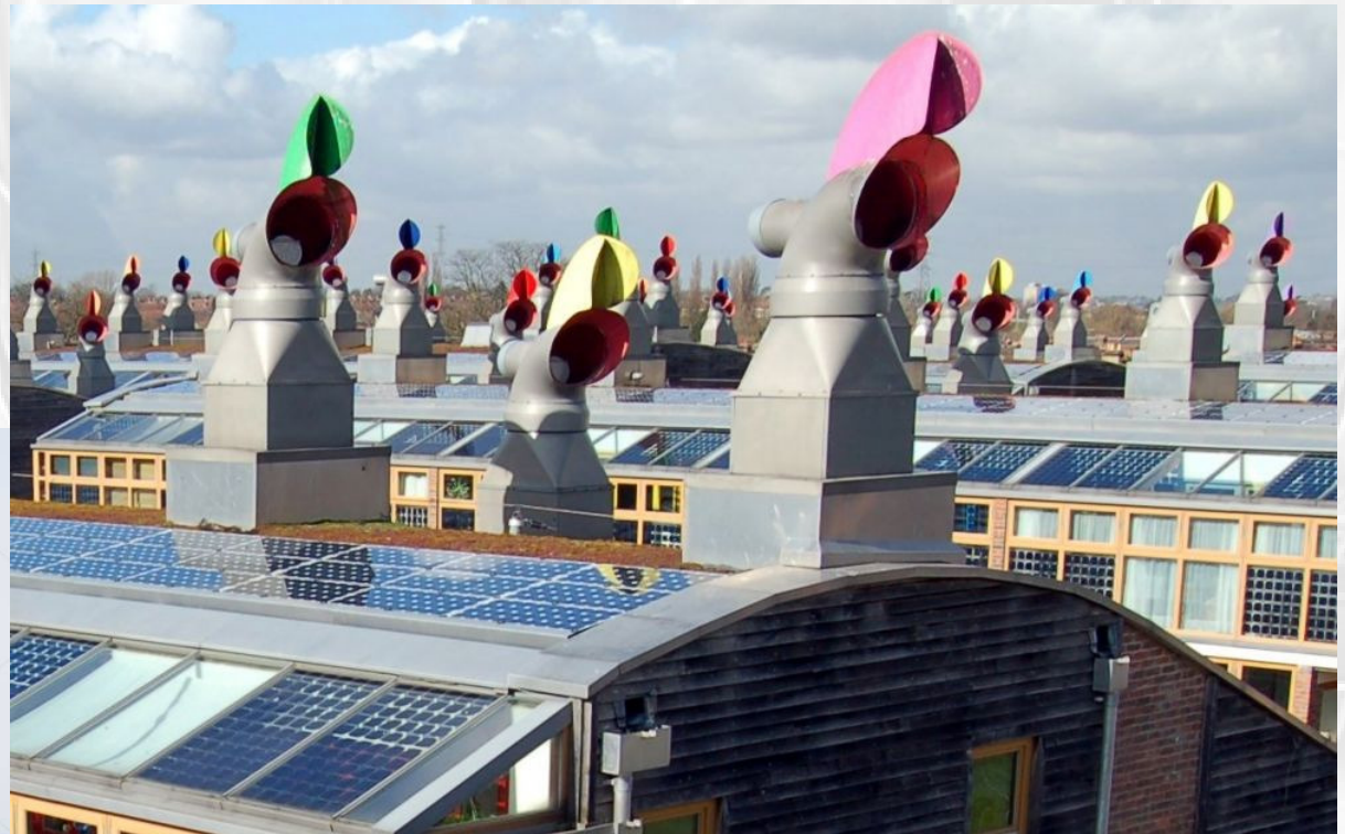
wind cowls in the BedZED development for passive ventilation
