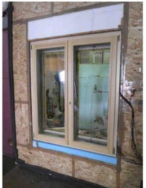
Fig. 16. – Window No. 2b – installed in the aperture of the surround panel
