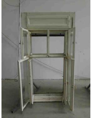
Fig. 12. – Window No. 1 – a typical early 20th century window with fix horizontal transom and a vertical mullion at the top (internal view)
