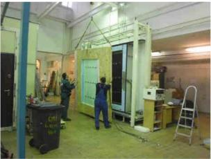
Fig. 8. – Hoisting the surround panel into place with the crane
