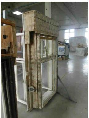
Fig. 13. – Window No. 1 – external view with the roller shutter case not having been removed jet
