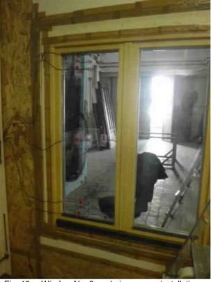
Fig. 19. – Window No. 2c – during sensor installation
