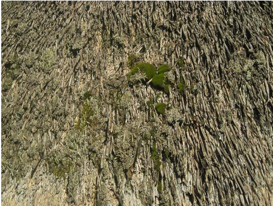
Moss and lichen on a thatched roof
