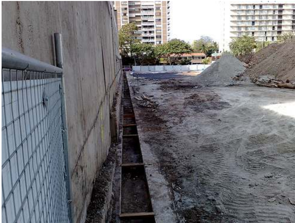
Alternatives for slurry wall guide walls
